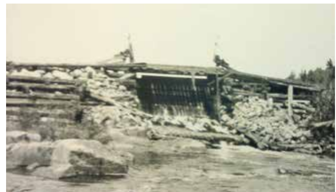
High Falls Dam
